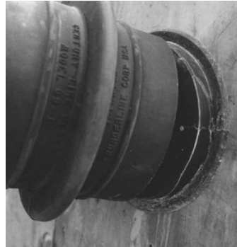
3. Place the Century-Line® Sleeve on the end cap. When field cutting non standard CS sleeve lengths, the sleeve and endcaps total length should be one-fourth (1/4") longer than the thickness of the wall. Cut with a hand or power saw. Note: To insure minimum water migration, center the water stop in wall by cutting equal lengths from each end of the sleeve, except as noted below.
