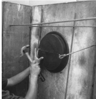
2. Nail one of the end caps at the marked center line.
