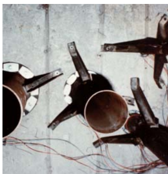
Certified test furnace with pipe and cable penetrations and fire rated Link-Seal® modular seal installed in concrete floor slab. Twenty-seven thermo couples were used per slab.
